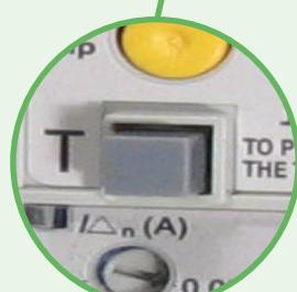
Test Button (to test the residual current detection and tripping system)
